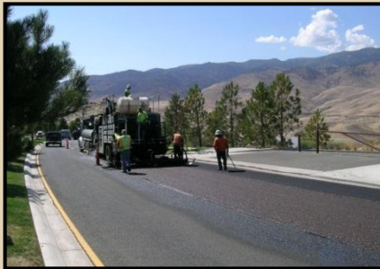
SLURRY SEAL TREATMENT
